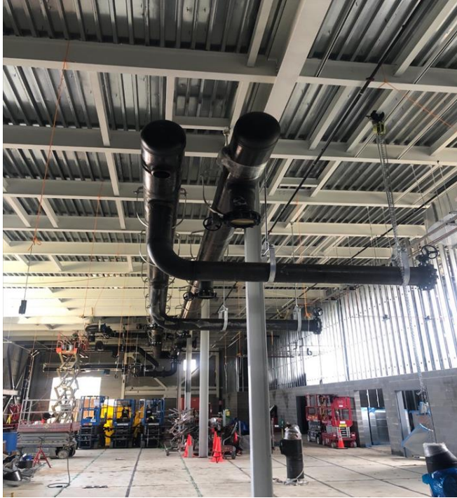
Geothermal weld prefab at WTCC CEP
